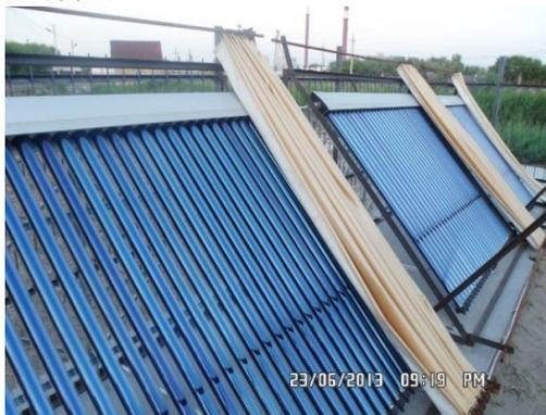
**Fig.1.** Solar system with a circulating intermediate coolant. Pilot plan
