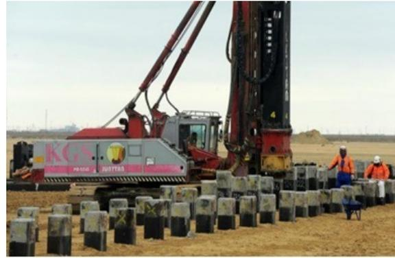
Fig. 4 Dynamic load testing in construction site on Tengiz
