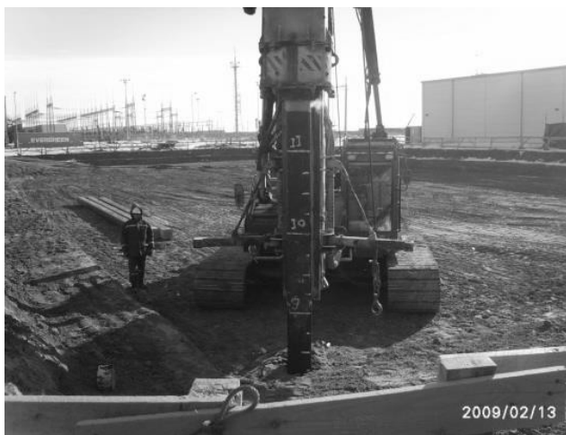
Figure 1. Dynamic test of pie driving by machine Junttan PM-25
