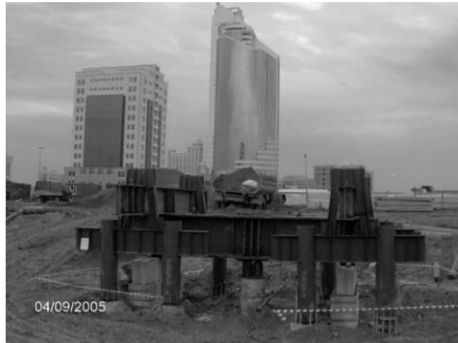
Figure 3. Static load test of bored pile performance
