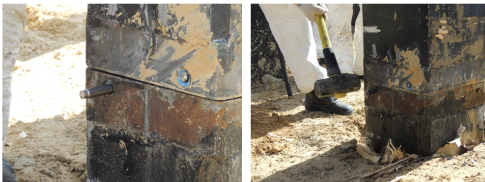
FIGURE 3 – Installation of two segments of precast concrete joint pile
