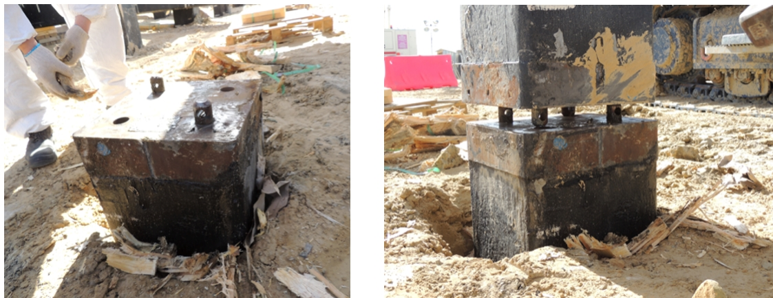
FIGURE 2 – Two female (socket) and two male (stud) locking mechanisms
